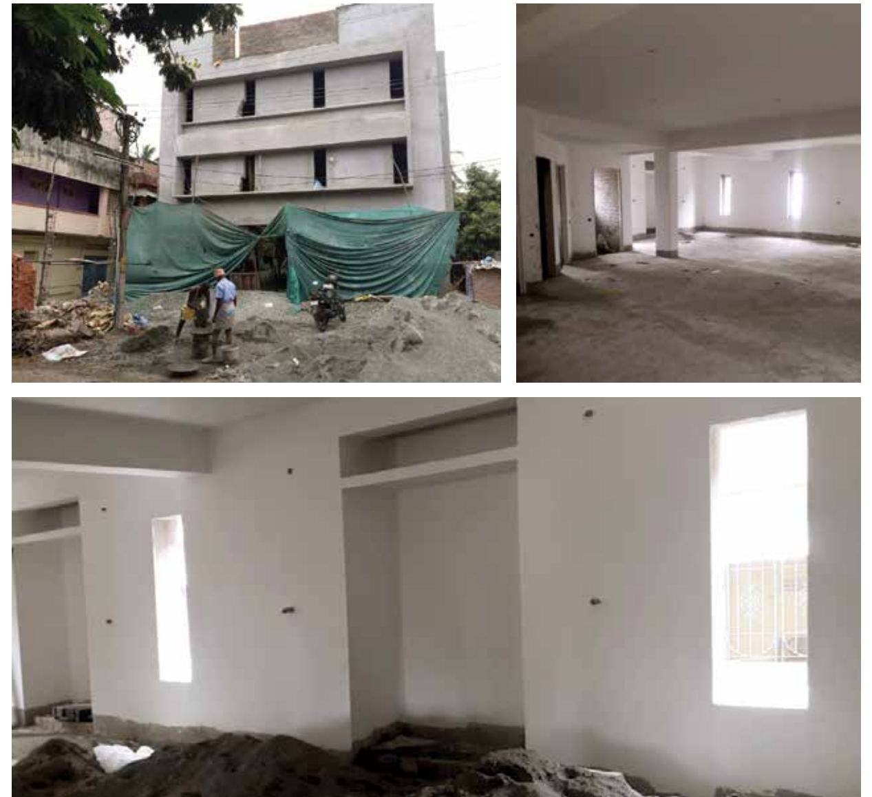
The dementia care inpatient facility in Tambaram, work in progress
